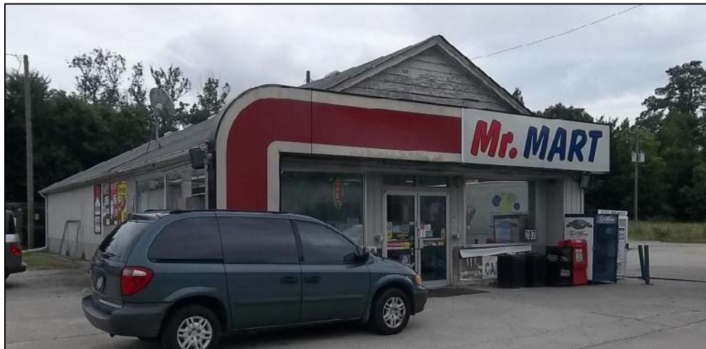
Photo 7: North Oblique, Office and Store/Mr. Mart Convenience Store.
