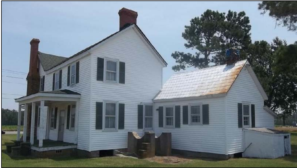
Photo 66: Northwest Oblique of the Rear Ell and the Kitchen.
