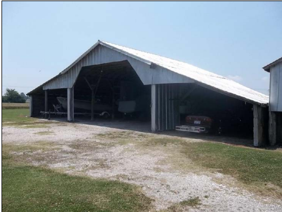
Photo 68: East Elevation of the Garage.
