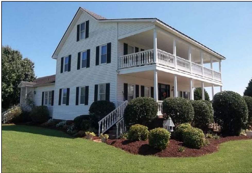
Photo 75: Detail of the Porch on the West Elevation.
