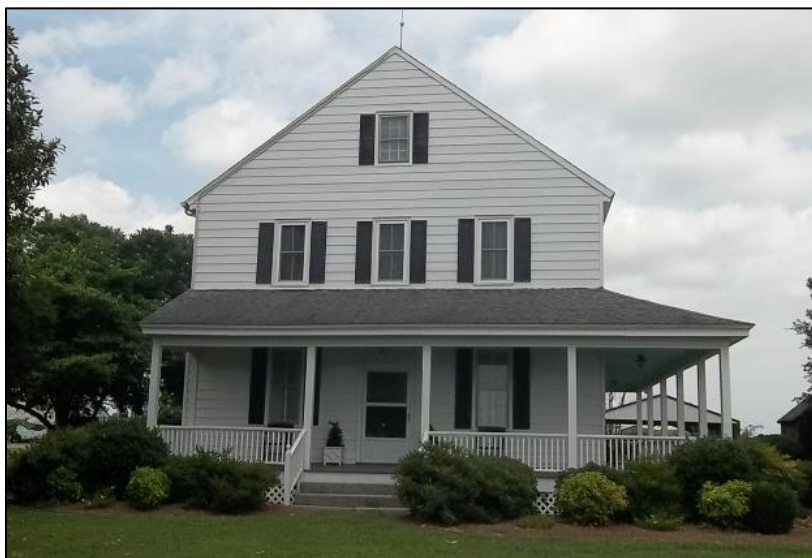
Photo 49: Primary Elevation of the John Humphries House; Similar in Form and Massing to Culong.
