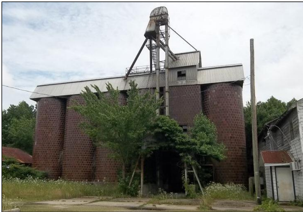
Photo 9: Northwest Elevation, Grain Elevator, Silos, and Loading Dock.
