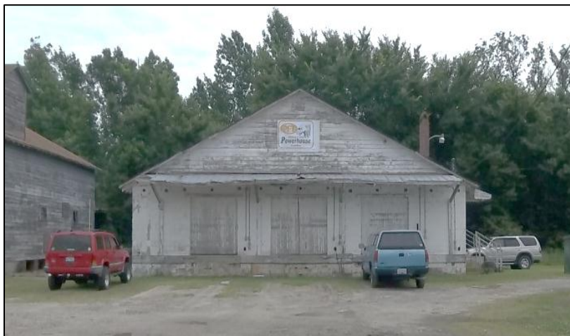
Photo 4: Northwest Elevation, Warehouse Two.
