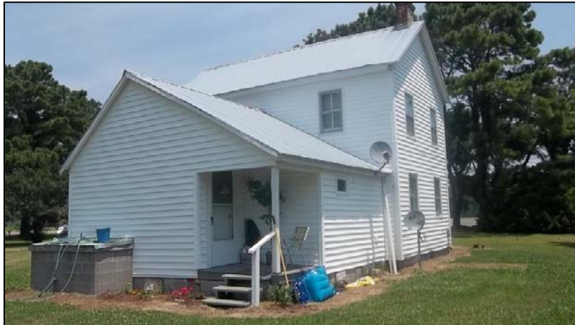
Photo 57: Southwest Oblique with a Detail of the Rear-Ell Addition.
