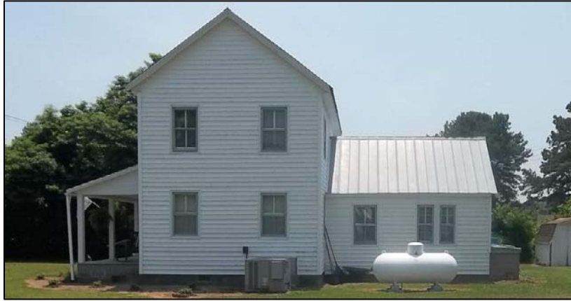
Photo 56: North Elevation of the Forbes House.
