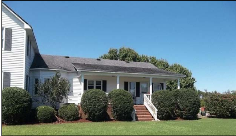
Photo 76: South Elevation of the One-Story Addition.
