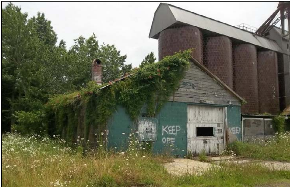
Photo 12: View of Warehouse Three/Garage, Looking South.
