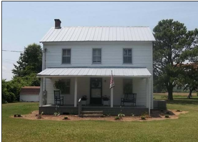
Photo 55: East Elevation of the Forbes House.
