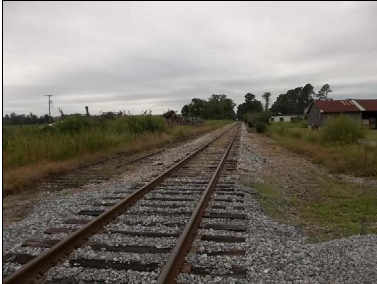
Photo 29: View of the Norfolk and Southern Railroad, Looking Southeast.
