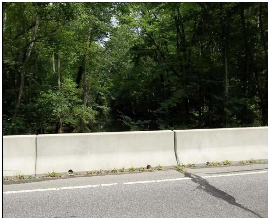
Photo 35: View of the Run Swamp Canal From U.S. Highway 158, Looking Northwest.
