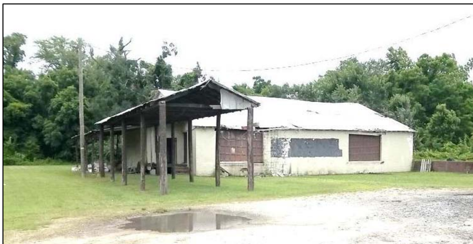
Photo 32: View of the Potato Grading Shed, Looking Northeast.
