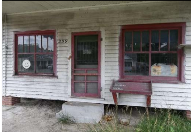
Photo 1: Detail of the Primary (Northwest) Elevation, Creekmore Store/Gas Station.
