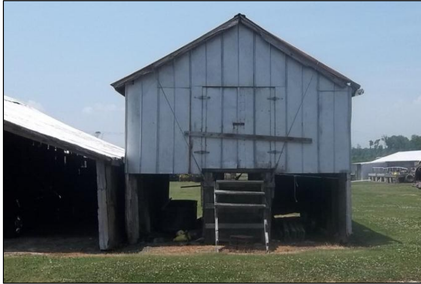
Photo 69: West Elevation of the Agricultural Outbuilding.
