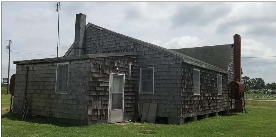
Photo 39: North (Rear) and West Elevation, Don Roberts House.
