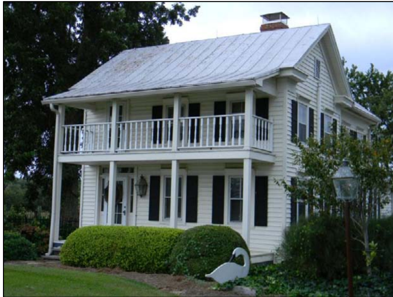
Photo 14: Detail of the Porch Located on the Northeast Elevation, Cooper House.
