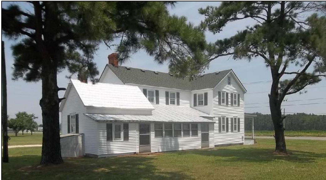
Photo 67: Southwest Oblique of the Forbes House, Rear Ell, and Kitchen.
