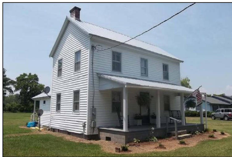
Photo 54: Southeast Oblique of the Forbes House.
