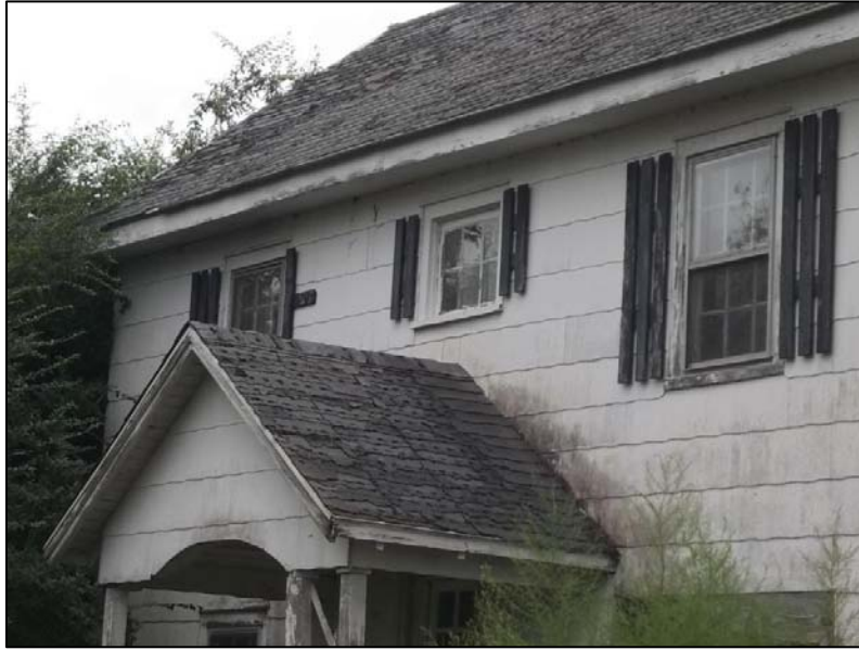
Photo 51: West Elevation, Second Story.
