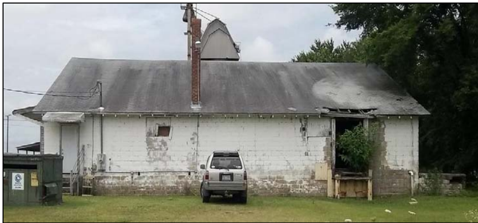
Photo 5: Southwest Elevation, Warehouse Two.
