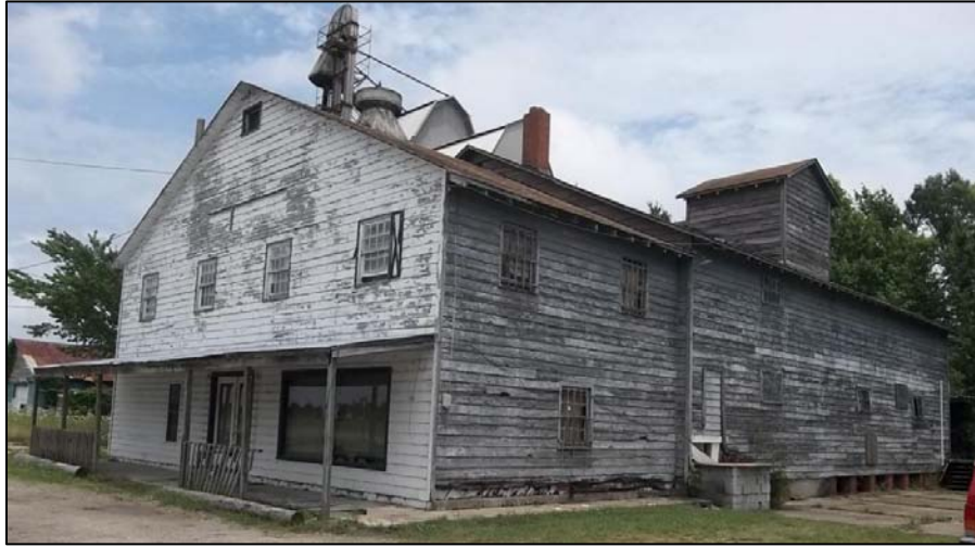
Photo 2: View of Warehouse One, Looking East.
