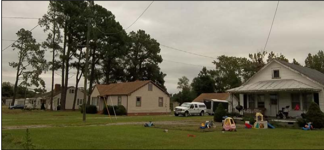
Photo 24: Overview of Houses Along U.S. Highway 158, Looking Northeast.
