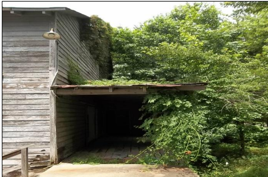
Photo 3: View of Loading Dock Looking Northeast, Warehouse One.
