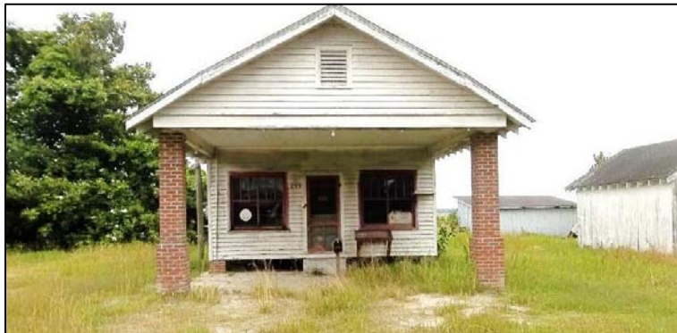
Photo 30: Northeast Elevation, Creekmore Store/Gas Station.
