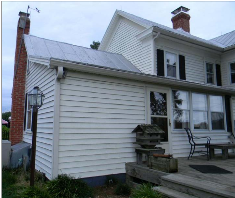
Photo 16: View of Kitchen Addition and Enclosed Porch, Looking North.
