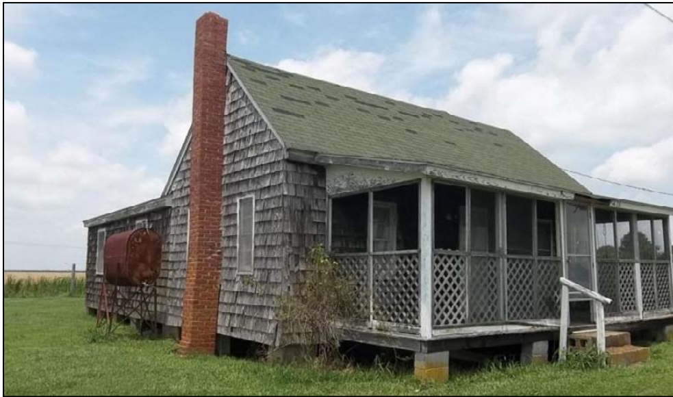
Photo 37: South (Main) and West Elevations, Don Roberts House.
