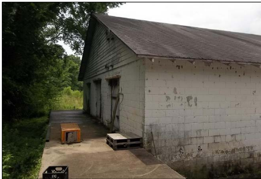
Photo 6: View of Southeast Elevation and Loading Dock, Warehouse Two.
