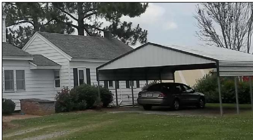
Photo 47: Second Carport, Southwest Oblique.
