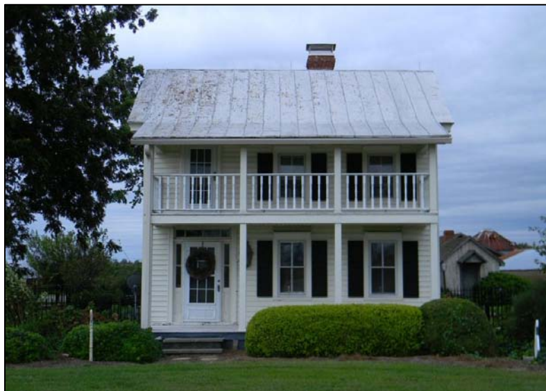
Photo 13: Primary (Northeast) Elevation, Cooper House.
