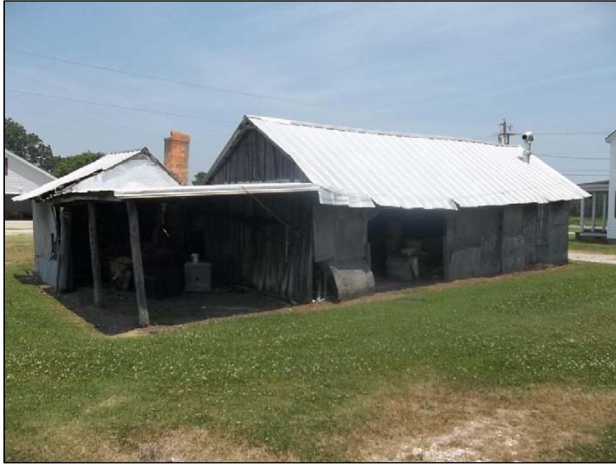
Photo 71: Southwest of the Shed/Workshop.
