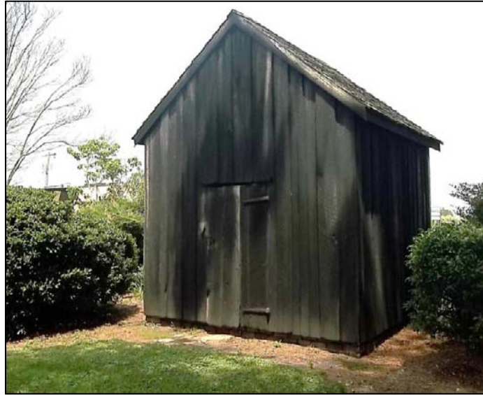
Photo 44: Smokehouse, Southwest Oblique.
